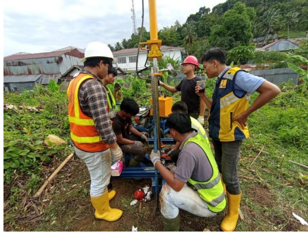
Figure 2. Cone Penetration Test Equipment
