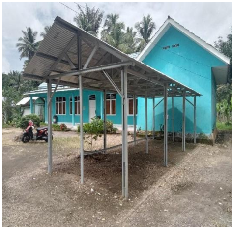
Gambar 1. Proses Pemasangan Paving 0%
